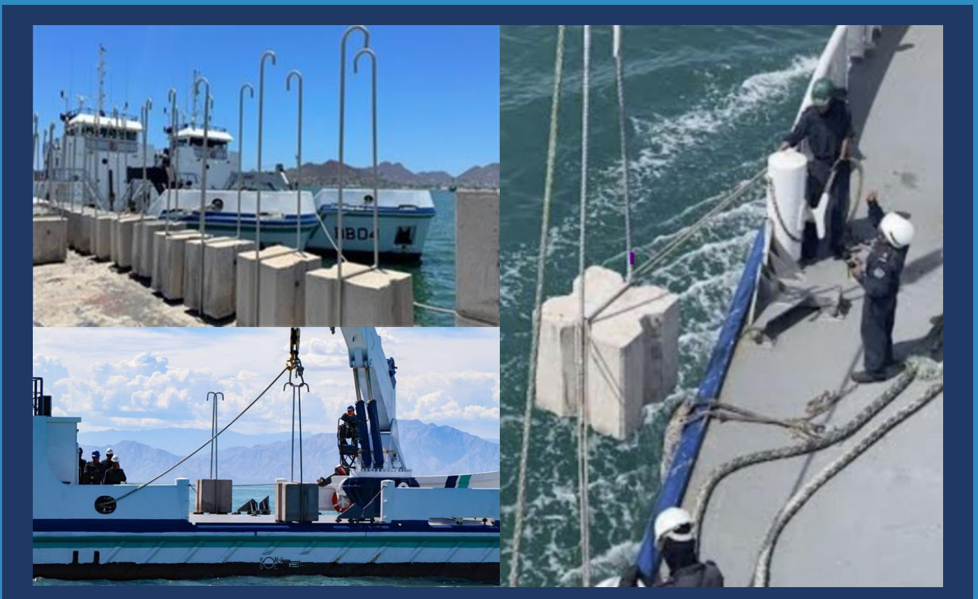
Figure 4: Deployment of anti-gillnetting devices made of concrete blocks with hooked rods, 3 meters high, that trap or entangle the nets on the seafloor of the Zero Tolerance Area (ZTA).
